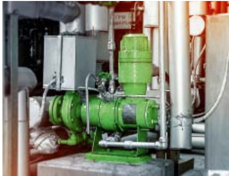
High-temperature type pump in a chemical plant.
