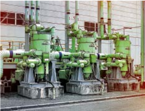
Reverse circulation type pumps for pumping LNG as Cooling medium. (Vertical type, Motor output 75kw)
